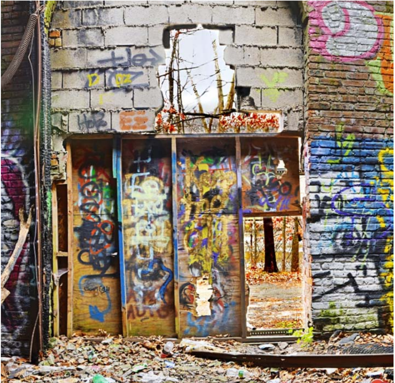
Figure 3.2. Consistent exposure between interior and exterior spaces.
